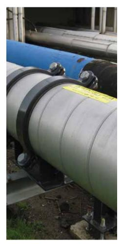
Pipe supports installed over the cladding guarantee uniform thermal profile along the entire pipe length.
