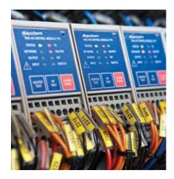
Central control and monitoring systems are typically installed in panels where they provide control and monitoring for several heat-tracing circuits or groups of circuits at the same time. They offer advanced features like measuring ground-fault levels, operating currents and provide a wealth of other maintenance-related information.
