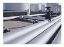
Applied to fluids that must be kept within a narrow temperature range to maintain viscosity and prevent fluid or pipe degradation. Typical examples include sulphur and acrylic acid lines.
